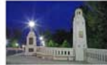
Lighting Restoration, Capitol Boulevard Bridge, Boise
