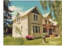
Front Porch Restoration, White Spring Ranch Museum, Genesee
