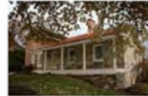
Exterior Restoration, Surgeon's Quarters, Fort Boise
