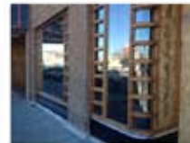
Glass Storefront Restoration, Romance Theater, Rexburg
