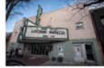
Exterior Tile Restoration, Kenworthy Theater, Moscow
